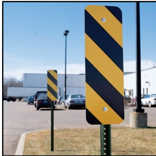
R27- Install delineators, reflectors, and/or object markers
