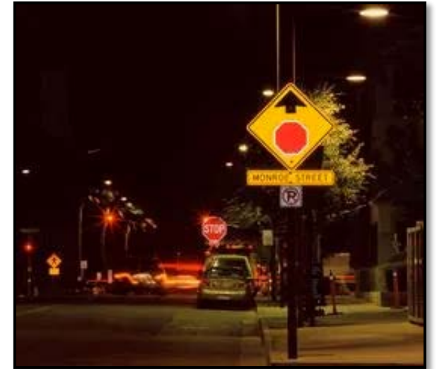
R22 - Install/Upgrade signs with new fluorescent sheeting (regulatory or warning)
